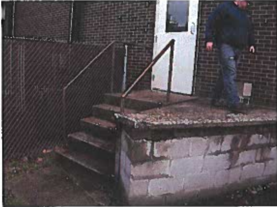
# 7 – Deck IMT Lab #8 – IMT Doors /Steps
