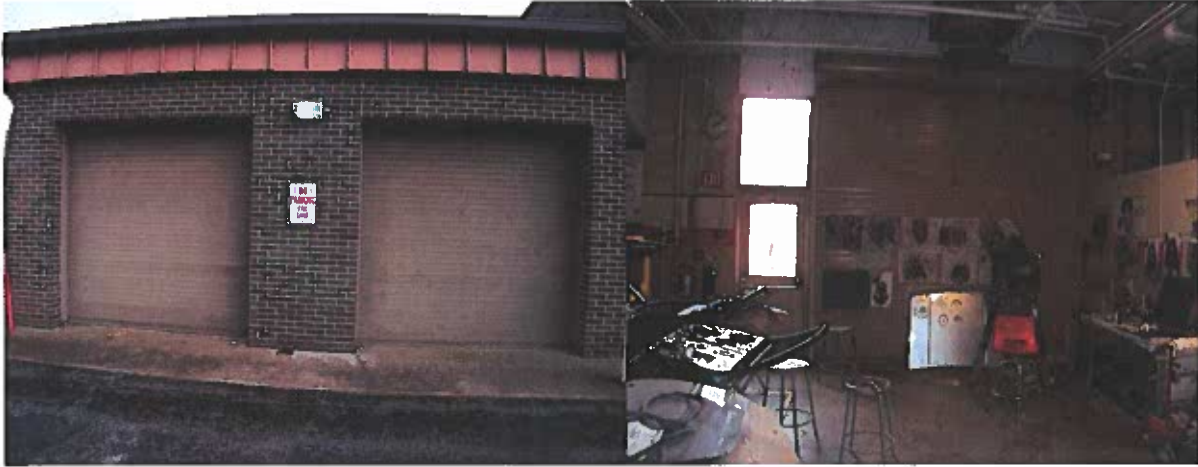
#12 – (3) Overhead Doors – Auto Collision Repair
